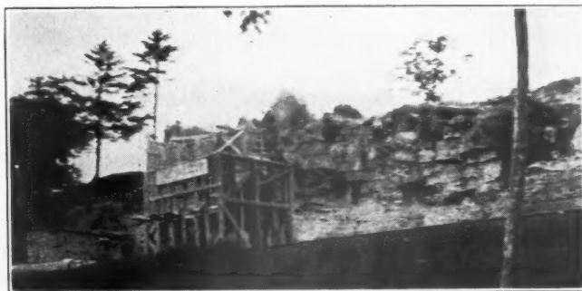
Setting Off the Blast at Lewiston
